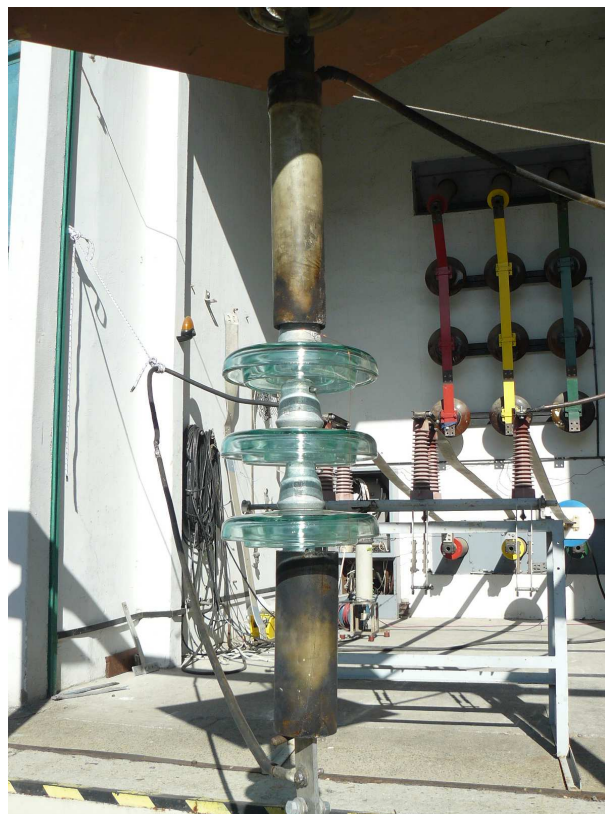
Photo 12 The first insulator string prepared for the power arc test
