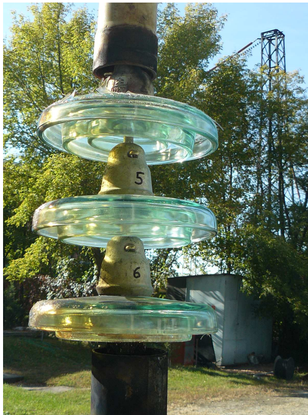
Photo 14 The second insulator string after the power arc test
